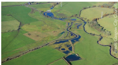
White Cart Flood Prevention Scheme achieved an overall 'Excellent' CEEQUAL rating with a score of 76.5%
