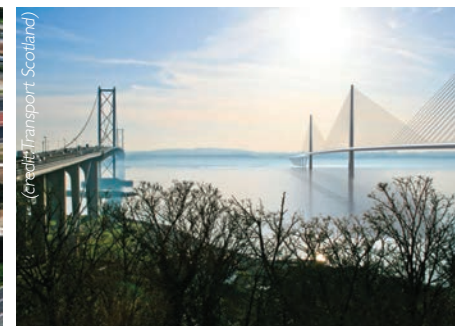
Forth Replacement Crossing achieved an overall 'Excellent' CEEQUAL rating with a score of 92.7%
