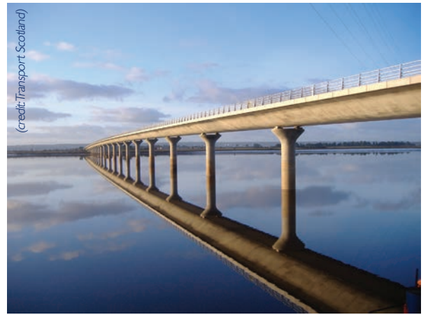
Kincardine Bridge - Forth Crossing achieved an overall 'Very Good' CEEQUAL rating
